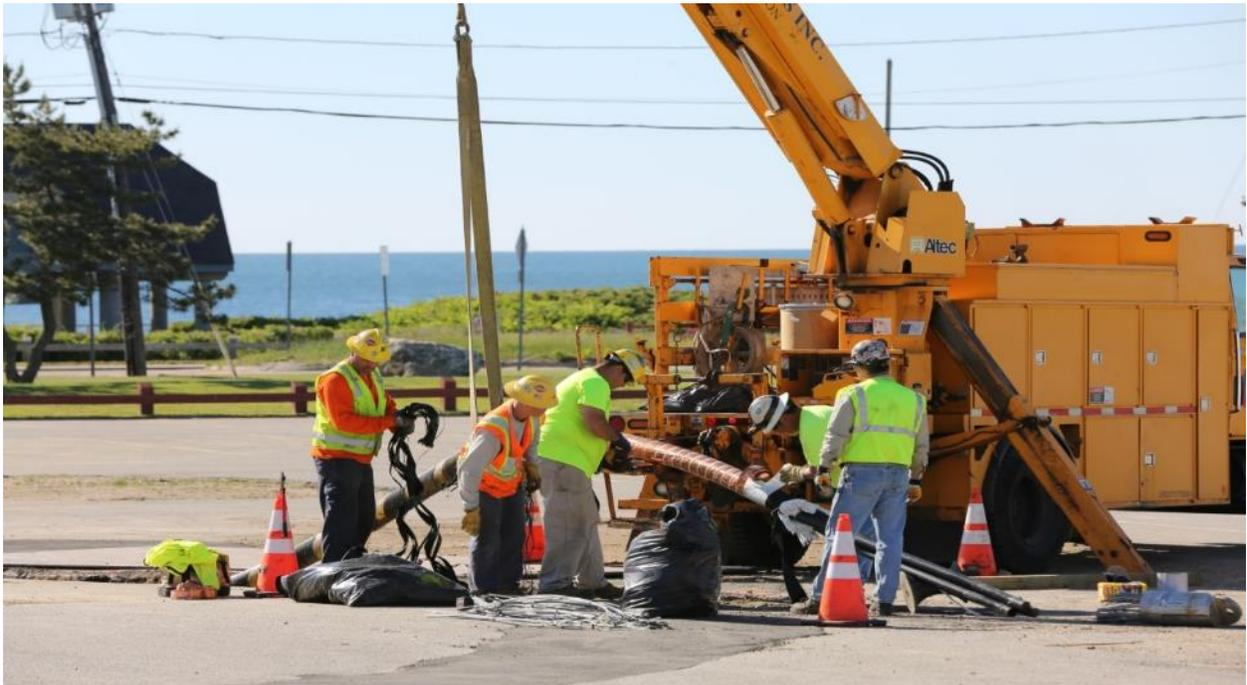
6/10/2016 Scarborough Beach State Park-Photo 0252: Stripping outer casing of BITS cable in order to splice into terrestrial cable.
