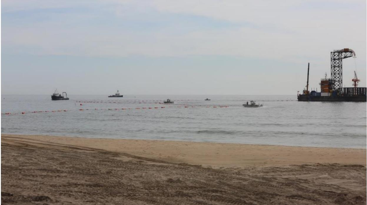
6/23/2016 Block Island Town Beach – Photo 0570: “Floating the cable”, orange buoys floating the remaining BITS cable to the surface in preparation for pulling to shore.
