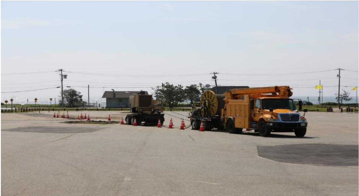
6/6/2016 Scarborough Beach State Park – Photo 0074: Utility truck, winch spool, and winch prepared for BITS cable pull to shore. The land sea transition vault is surrounded by cones.
