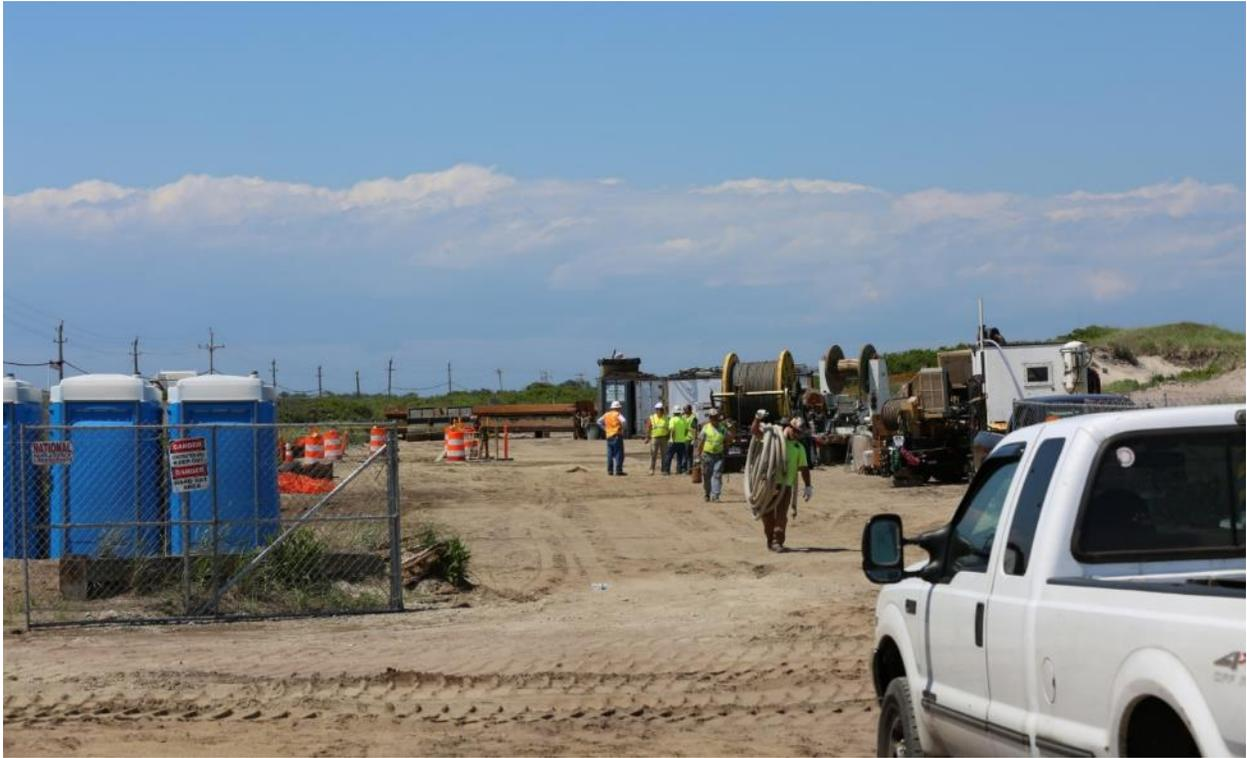
**6/22/2016 Block Island Town Beach – Photo 0513: Construction area west of sand dune located north side of Fredrick J. Benson Pavilion adjacent to Corn Neck Road. Winch spool and winch visible used for pulling BITS to shore. Orange barrels surround land sea transition vault.**
