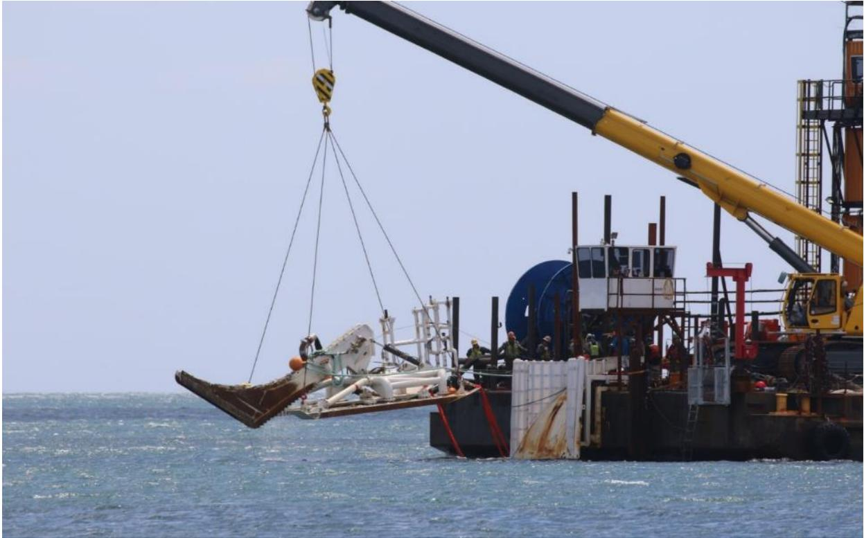
6/9/2016 Scarborough Beach State Park – Photo 2740: Jet Plow being lowered into the water aft of CLB Big Max.
