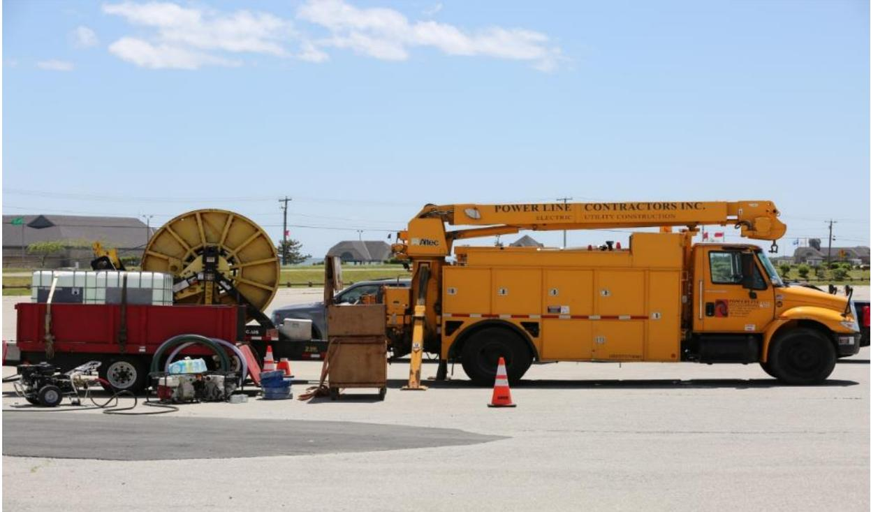
6/9/2016 Scarborough Beach State Park – Photo 0171: Cable pull initiation. Utility truck, winch spool, trailer with water and pressure washer used to spray salt water off the winch cable upon retrieval.
