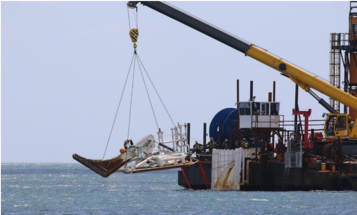
Figure 4. Jet Plow being lowered into water
