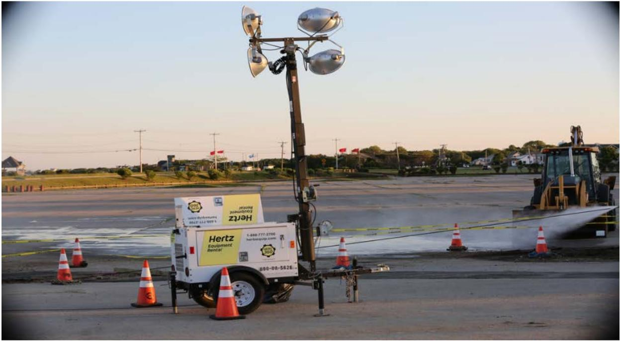
6/9/2016 Scarborough Beach State Park – Photo 0207: Portable lighting brought to site around dusk during cable pull. The winch cable is being washed as it is pulled back into shore.
